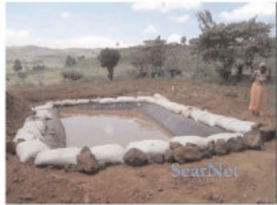
Plastic lining anchored with sand-bags
