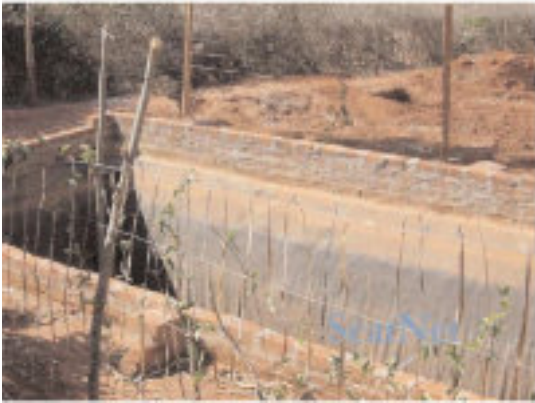
Plastic lining anchored with brick wall:
